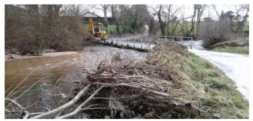
Clearing Debris from bridge for structural assessment.
