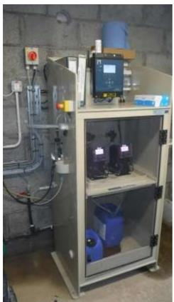
The new all-in-one chlorination cabinet, a trial unit which was designed by staff and constructed for use at the Ballyloo secondary chlorination site.
