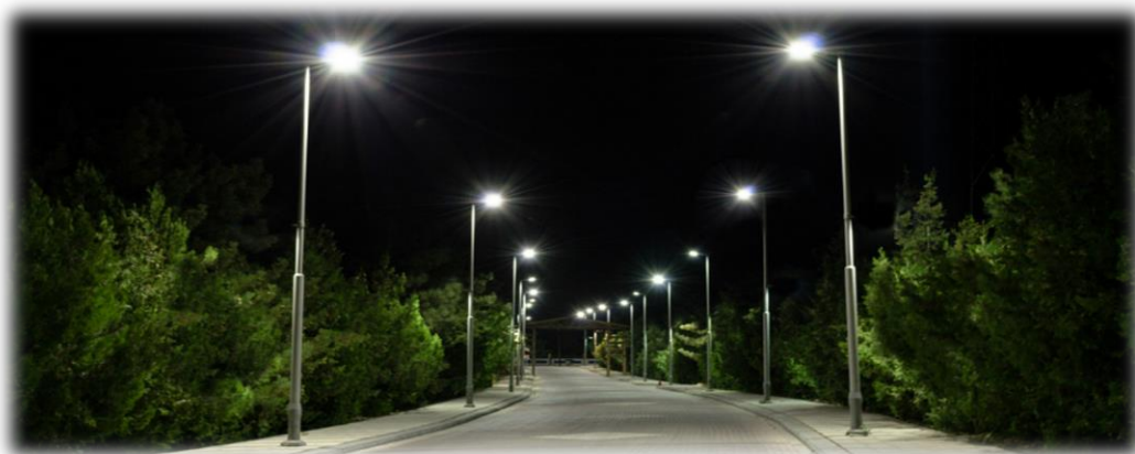
Figure 5.14 Carlow Public Lighting Efficiency Project
