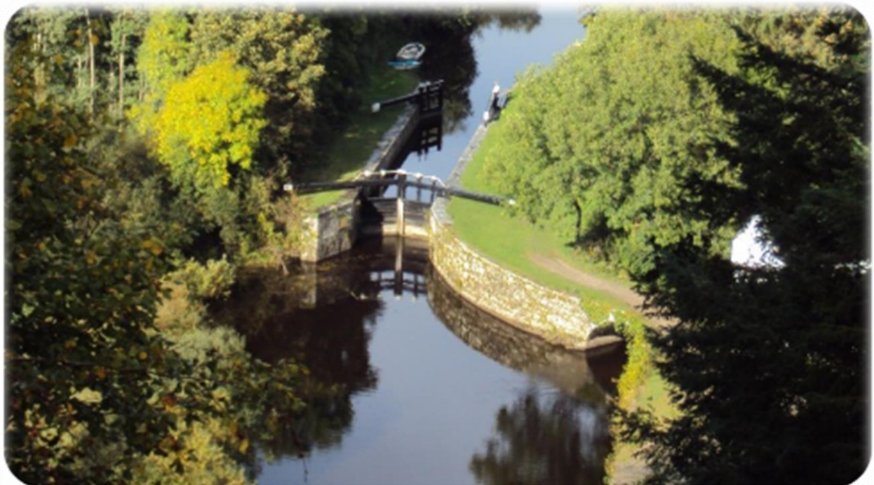
Figure 2.3 Clashganney Lock, Borris , Co. Carlow.
