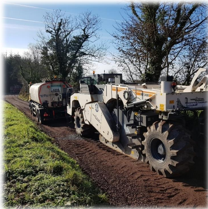
Figure 2.12 Road Recycling in Staplestown, County Carlow
