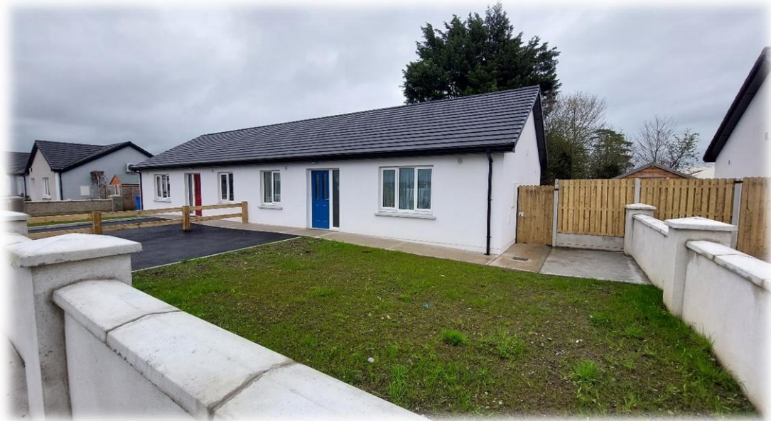
Figure 5.19 H4.0E Pilot in St Mary's Court, Carlow Town
